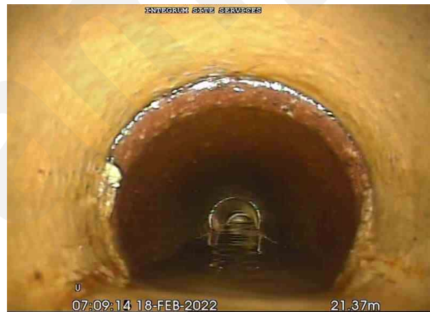
1-1-13A, 00:02:51, 21.57 m Pipe material changes to vitrified clay at this point, 21.57
