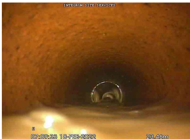
1-1-14A, 00:03:10, 23.42 m Survey abandoned, Camera unit goes underwater and loses vision
